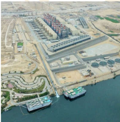
New Capital Power Plant
