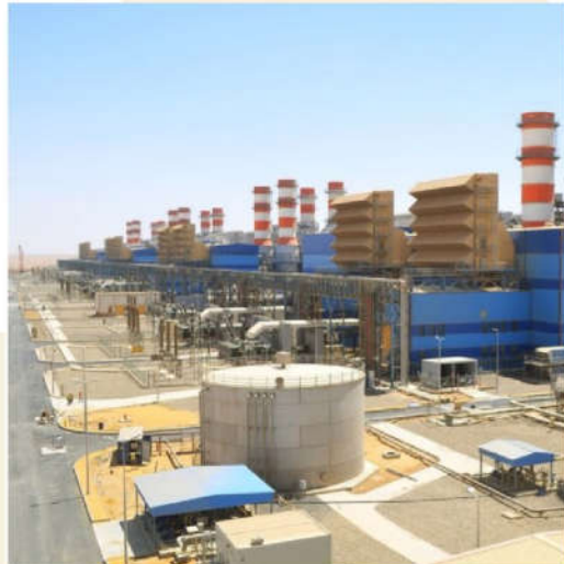
Beni Sueif Power Plant
