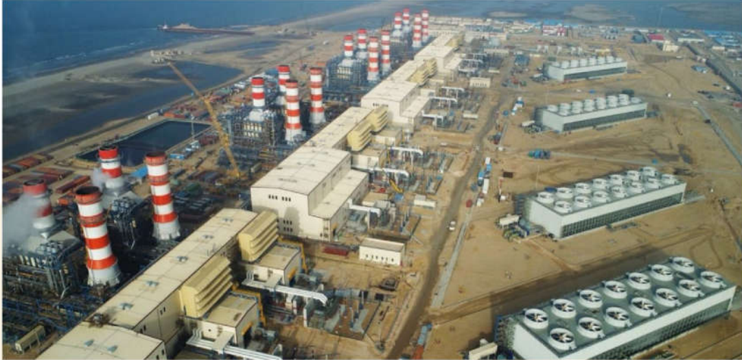
Burullus Power Plant
